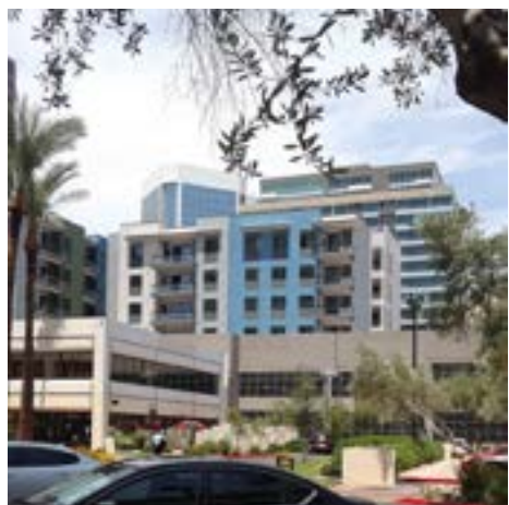
Edison Midtown Condos 3131 N Central – joins the northwest-looking skyline between the Great American Tower, 3300 N Central Ave and One Lexington
